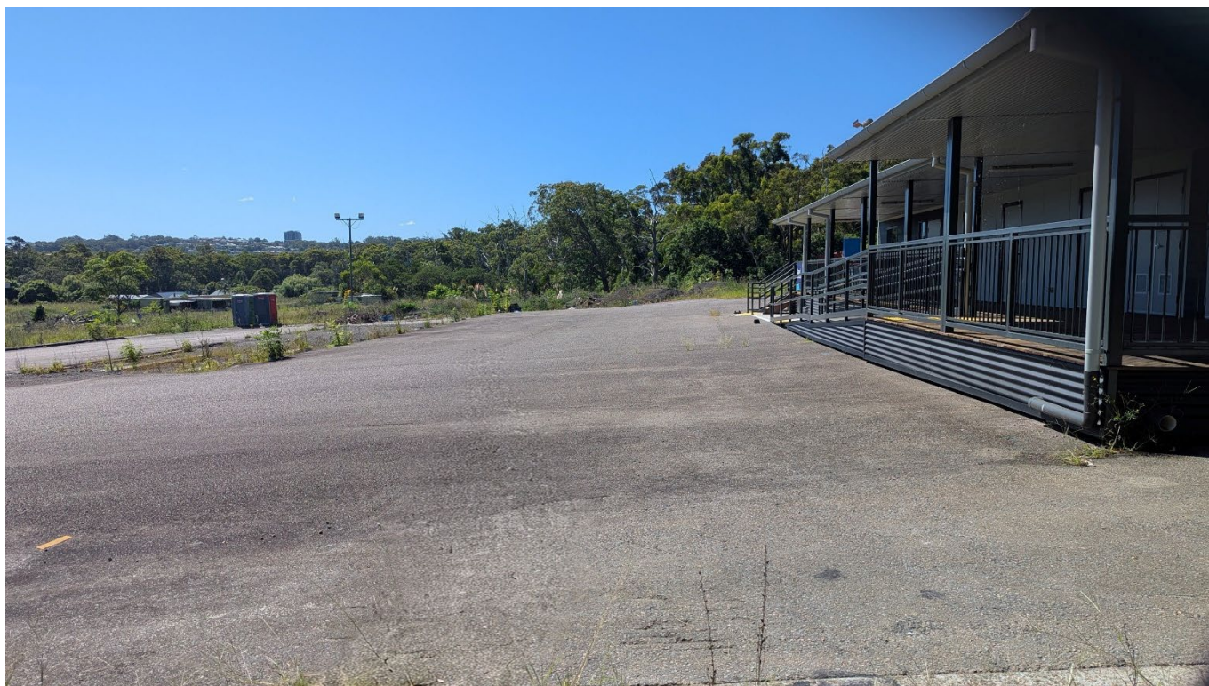
Figure 8 – Existing vacant Transport for NSW structure on the site adjacent to the development site
