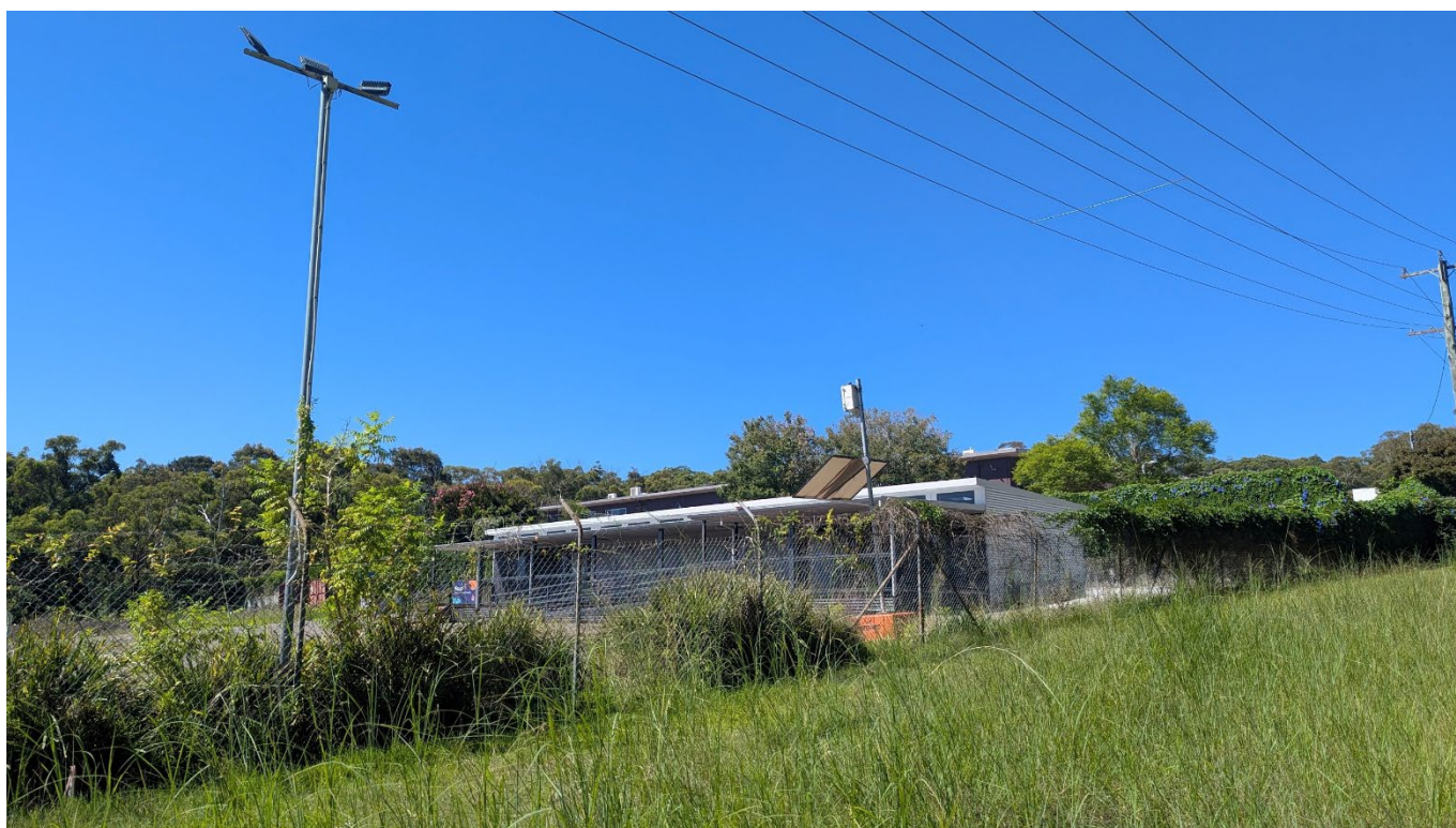
Figure 7 – Existing vacant Transport for NSW structure on the site adjacent to the development site
