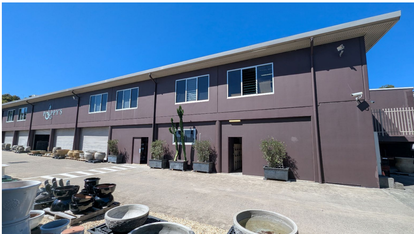
Figure 10 – Existing development to the immediate east of the Transport for NSW depot site – Poppy's Home and Garden Centre
